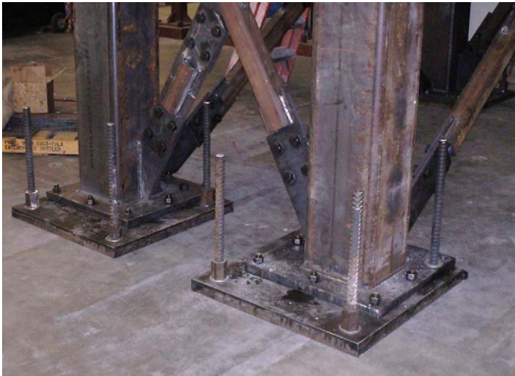
Figure 2. Test structure connection to the LAB site strong floor.
