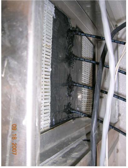
Underneath the new valve/dipper assembly there is a trough with a drain tube to outside the building (the drain tubes runs outside where the blue, flexible vent air hose from the cooler penetrates the wall to the right of the battery inclosure). Any leaks from the assembly should be caught by the trough and drained to the outside. A Plexiglas door in front of the assembly should divert and 'spraying' leaks down to the trough.
