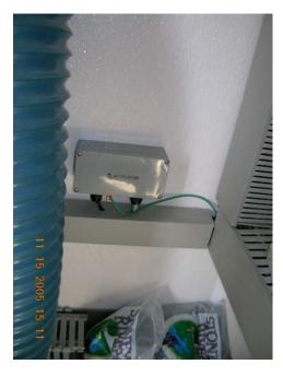
Power-injection for the WiLan VIP-110 radio (mounted on the roof adjacent to the parabolic antenna) is done in the lightning protection box mounted above the horizontal caterpillar on the back-wall of the hut to the right of battery enclosure.
