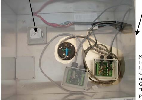
NOTE: The cabling from the sensor to the LP board in the wellhead box uses colorcodes from the legacy GVDA wiring where "black" was the positive!
