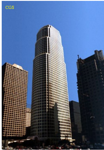
Figure 3.1. Los Angeles 54 story office building
