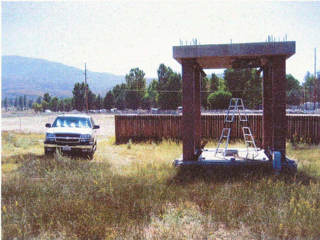
General Site View
