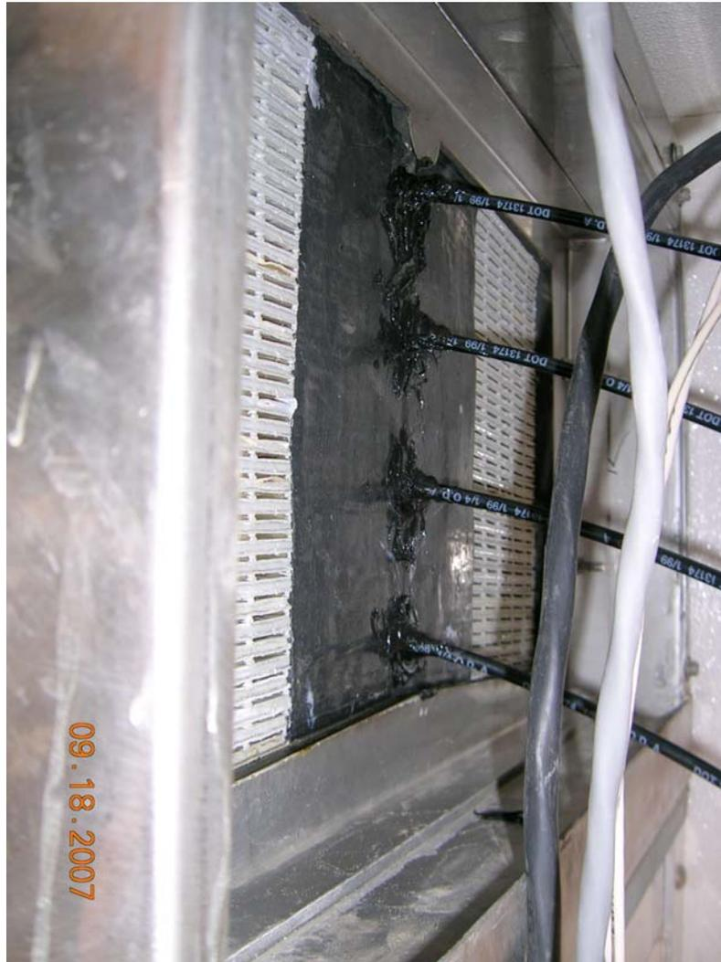
Underneath the new valve/dripper assembly there is a trough with a drain tube to outside the building (the drain tubes runs outside where the blue, flexible vent air hose from the cooler penetrates the wall to the right of the battery inclosure). Any leaks from the assembly should be caught by the trough and drained to the outside. A Plexiglas door in front of the assembly should divert and 'spraying' leaks down to the trough.
